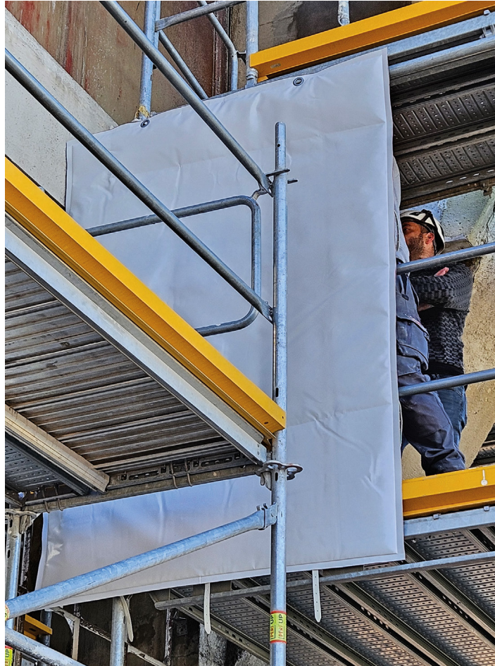
Fig. 2: Start of installation, alignment
