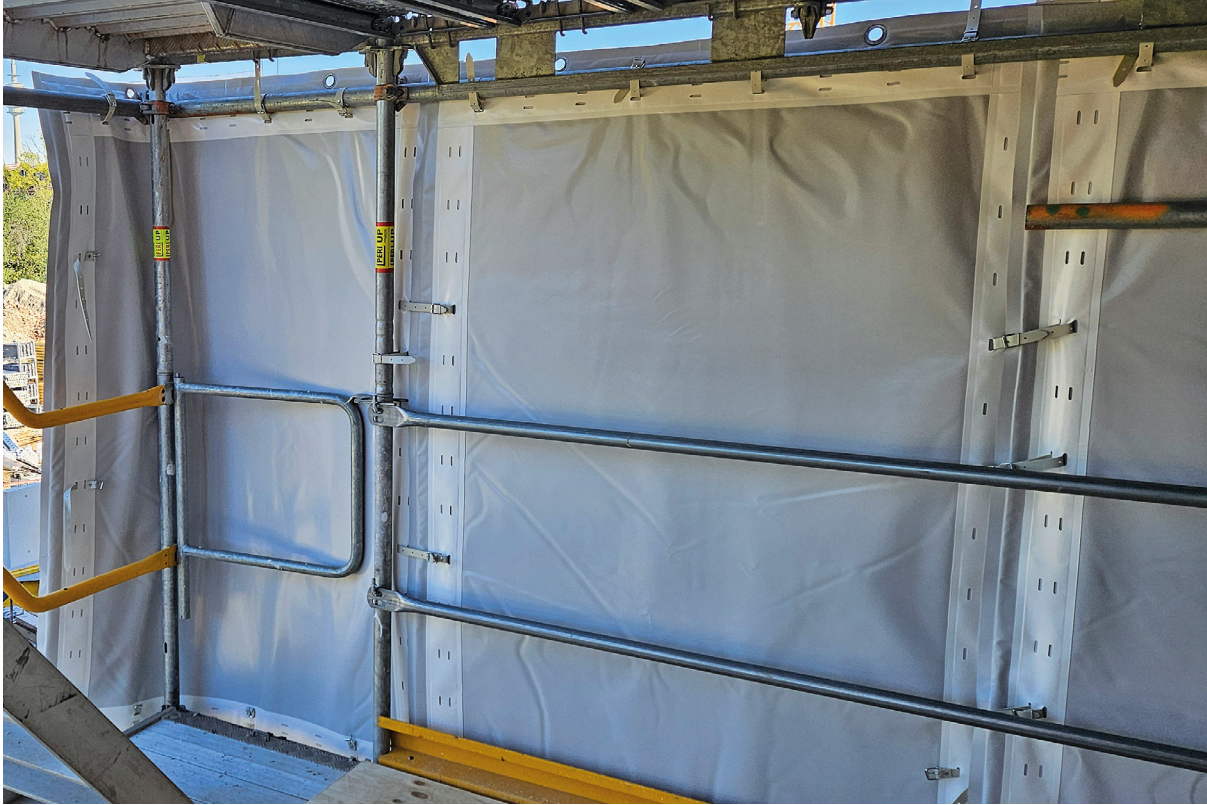
Fig. 4: Fastening to vertical scaffolding pole, connection of Cisilent in middle of section
