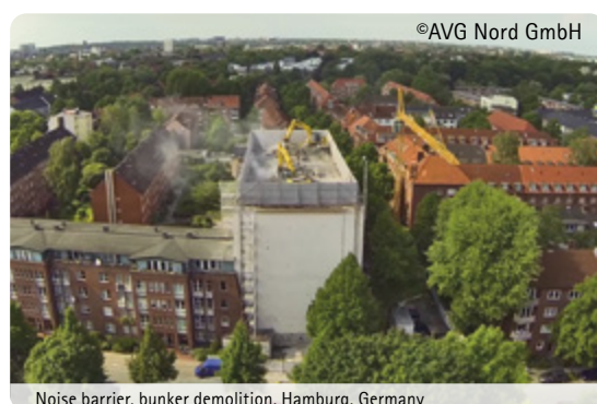
Noise barrier, bunker demolition, Hamburg, Germany
