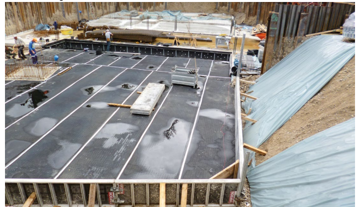
Residential buildings in Bauseweinallee, Cibatur® installed in one and two layers
