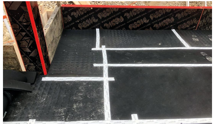
Single-family houses in Gräfelfing, installation of Cibatur® in one and two layers under the foundation
