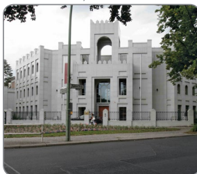
Qatar Embassy Residence (DE)
