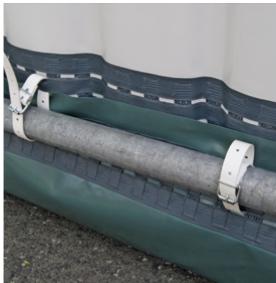
Figure 8: Fastening protective strip to scaffolding pole
