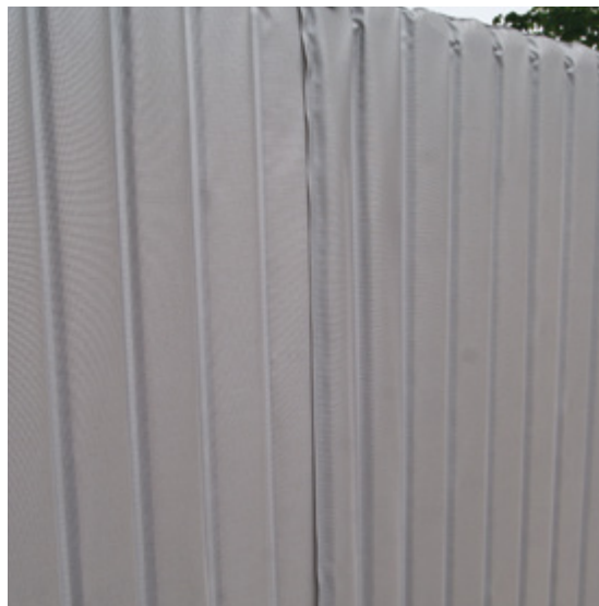
Figure 6: Edges overlap to provide a seal
