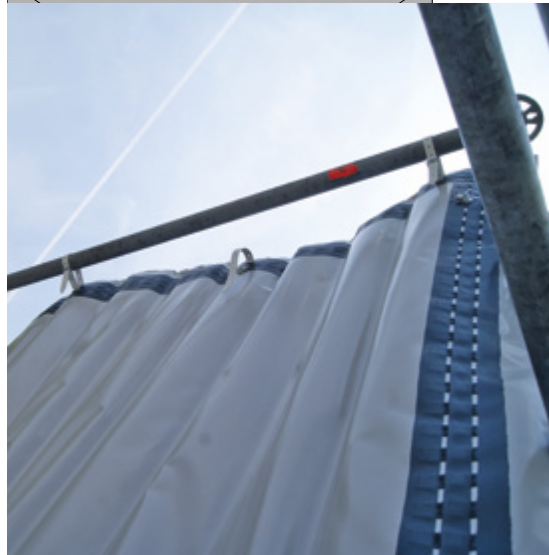
Figure 4: Fastened and aligned
