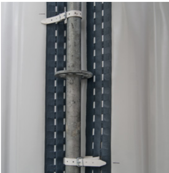
Figure 5: Alignment, fastening to the scaffolding post
