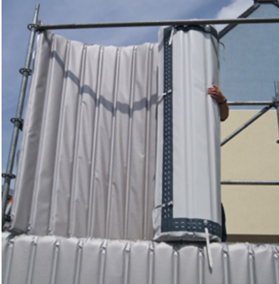
Figure 3: Unrolled in a scaffolding section
